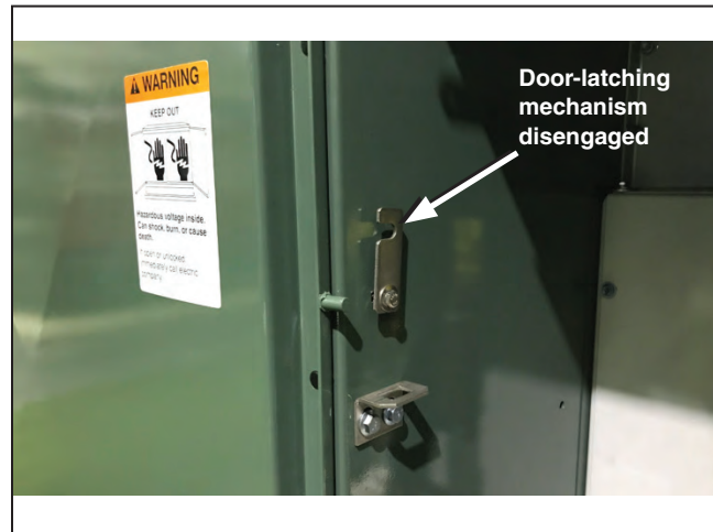
Figure 5. The left-door latching mechanism disengaged.
