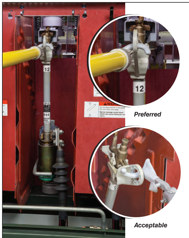
Figure 26. A Grappler tool, as positioned for an opening stroke.
