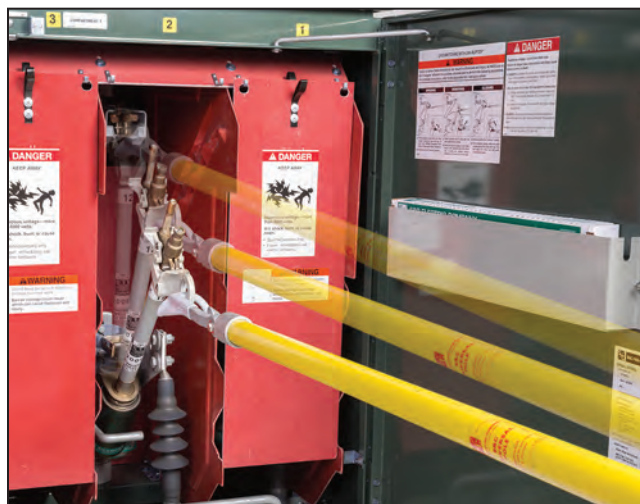
Figure 27. Opening the fuse.
