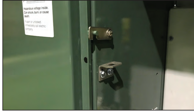
Figure 9. The left-door latching mechanism engaged.
