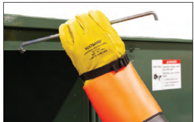
Figure 7. Lift the door holder to allow the door to swing closed.
