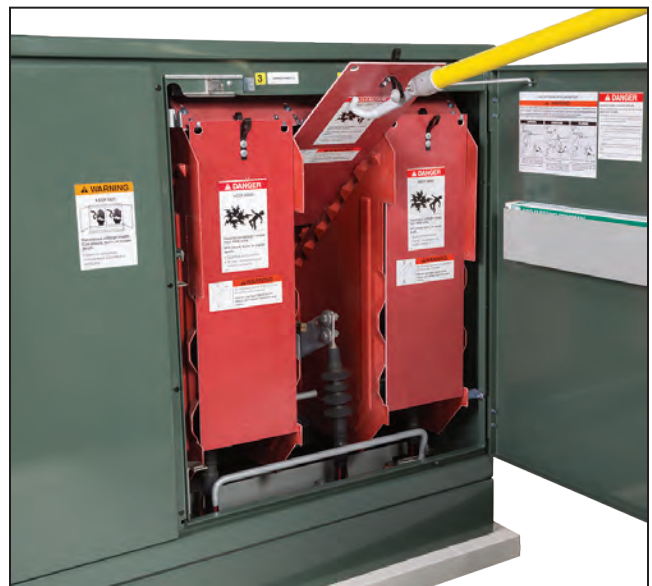
Figure 21. Inserting the dual-purpose front barrier into the Slide In position using a Grappler tool.
