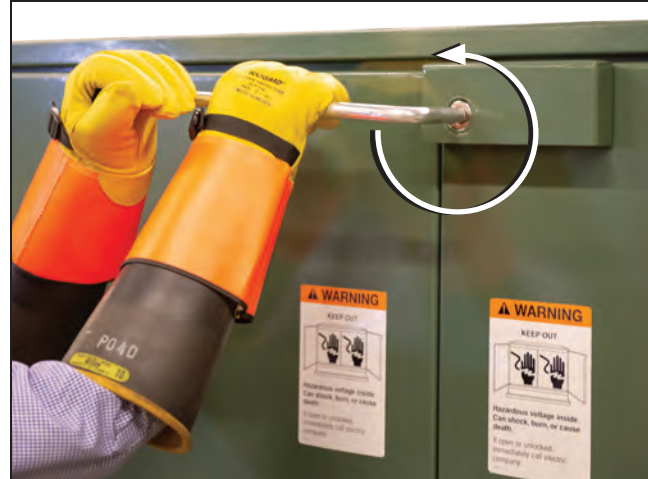
Figure 4. To unlock the doors, turn the pentahead socket wrench 60° counterclockwise against spring resistance until a “click” is heard and the wrench reaches its stop.
