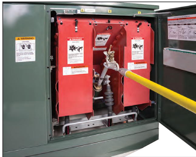
Figure 23. A fuse installed in mounting in the Open position.
