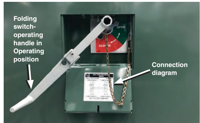
Figure 13. The switch operating handle installed.
