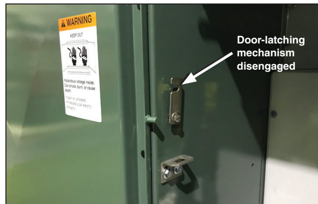
Figure 5. Rotate the latch upward to disengage the left-hand door, as shown above. To secure the left-hand door closed, rotate the latch downward over the stop on the outer edge of the door.
