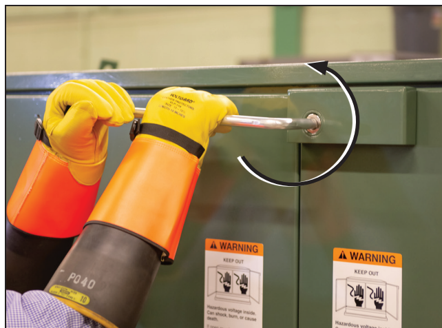
Figure 3. To unlock the doors, turn the pentahead socket wrench 60° counterclockwise against spring resistance until a “click” is heard and the wrench reaches its stop.
