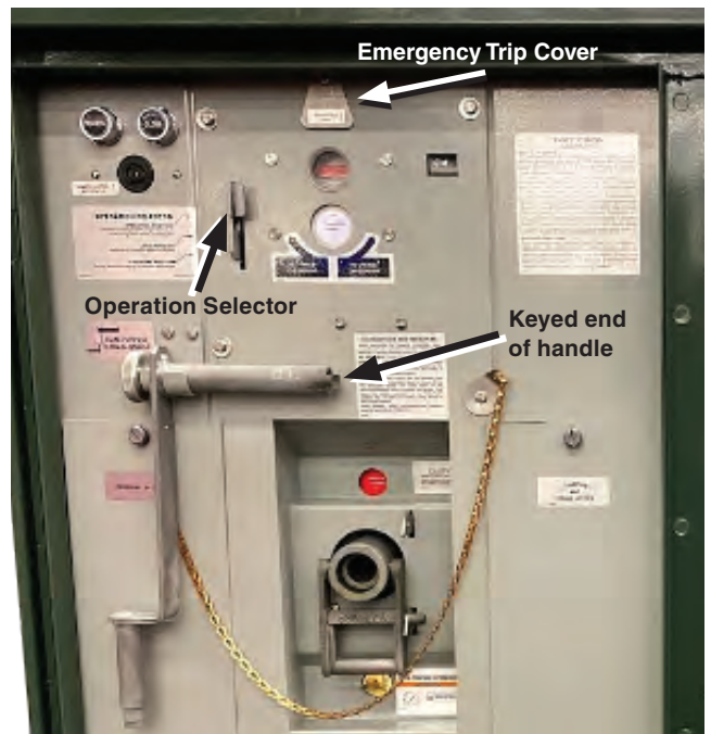
Figure 13. The keyed end of the dual-purpose manual handle can be inserted into the groove of the tripping shaft for emergency manual switching if control power is lost.
