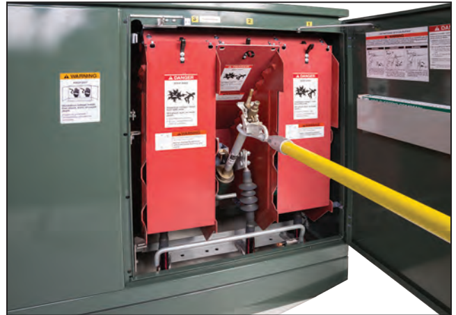
Figure 23. A fuse installed in the mounting in the Open position.
