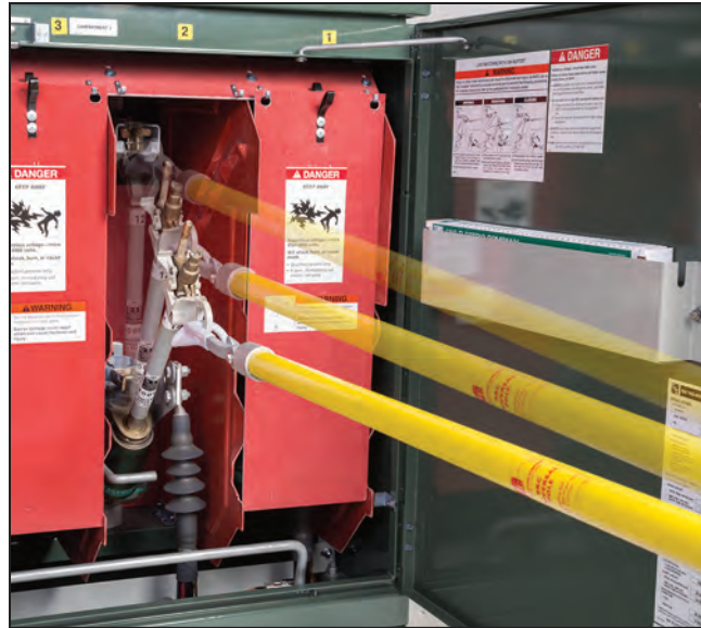
Figure 27. Opening the fuse.
