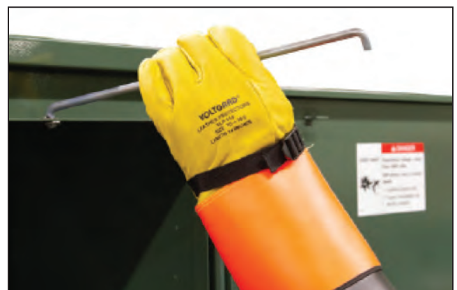
Figure 8. Lift and store the door holder to allow the door to swing closed.
