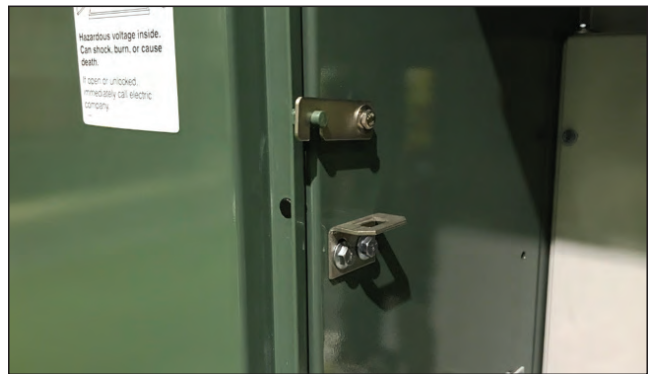
Figure 10. The left-door latching mechanism engaged.
