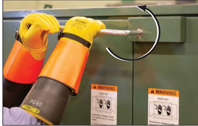
Figure 5. To unlock the doors, turn the pentahead socket wrench 60° counterclockwise against spring resistance until a “click” is heard and the wrench reaches its stop.
