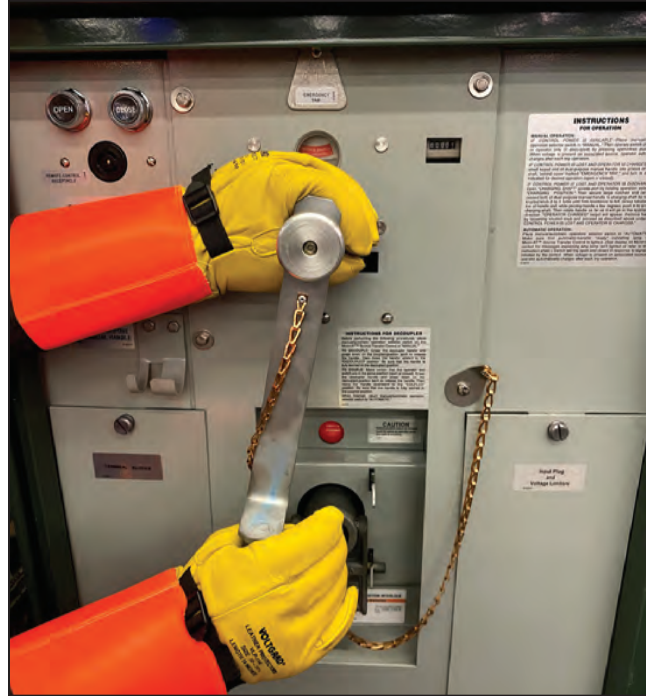
Figure 14. Dual-purpose manual handle on the charging shaft.
