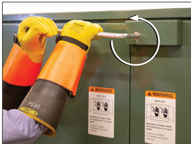
Figure 2. To unlock the doors, turn the pentahead socket wrench 60° counterclockwise against spring resistance until a “click” is heard and the wrench reaches its stop.
