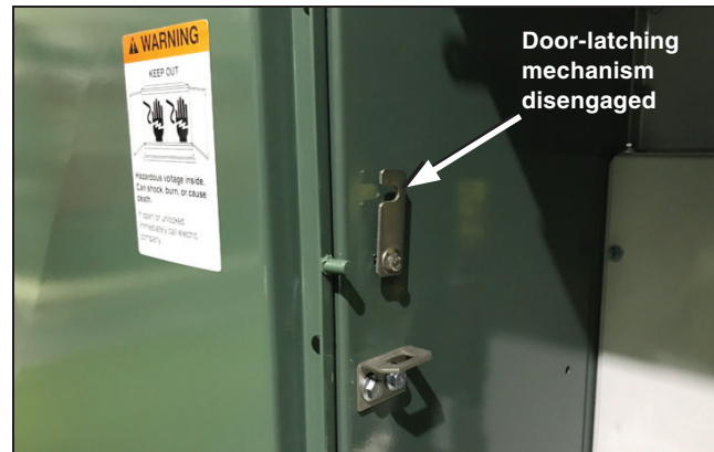
Figure 4. Rotate the latch upward to disengage the left-hand door, as shown above. To secure the left-hand door closed, rotate the latch downward over the stop on the outer edge of the door.
