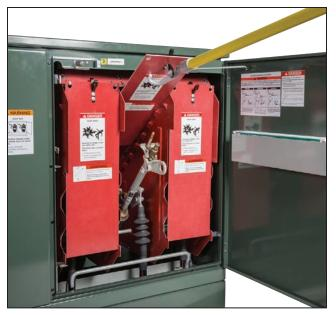
Figure 27. Inserting dual-purpose front barrier into the "slide-in" position using a Grappler tool.
