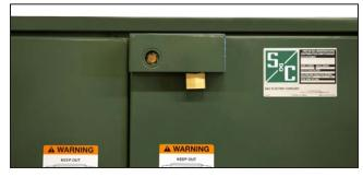
Figure 9. The enclosure doors padlocked.
