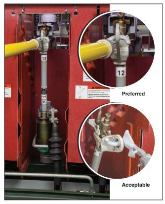
Figure 25. Grappler tool, as positioned for an opening stroke.
