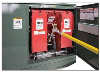
Figure 22. A fuse installed in mounting in the Open position.
