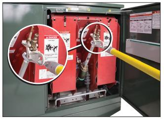
Figure 21. Installing a fuse using a Grappler Handling Tool. The inset image shows a close-up of a Grappler tool in position to install the fuse.
