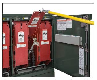
Figure 23. Removing dual-purpose front barrier from the "Slide-in" position using a Grappler tool.
