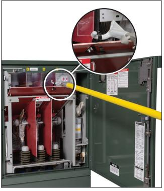
Figure 16. The Grappler tool, after lifting and pivoting the barrier, is used to lower it into the Slide In position. The image also shows the Grappler tool being used to return the barrier to its normal, suspended position.
