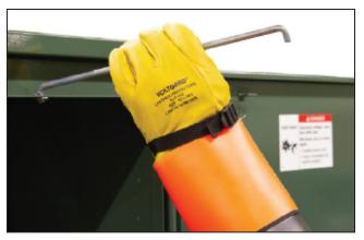
Figure 6. Lift the door holder to allow the door to swing closed.
