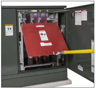
Figure 15. A Grappler Handling Tool being used to lift the barrier. Note the door holder is in place and the adjacent door is latched closed to reduce exposure to high voltage.
