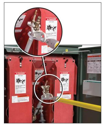
Figure 28. A Grappler tool positioned for fuse removal.
