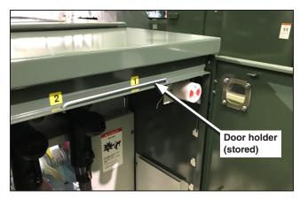
Figure 7. The door holder placed in the storage position to allow the door to close.
