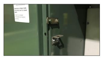
Figure 8. The left-door latching mechanism engaged.
