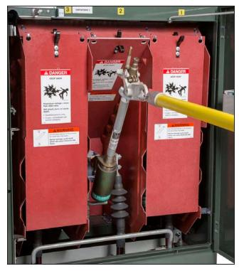
Figure 29. Removing a fuse from its hinge with a forward and upward lifting motion.
