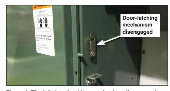
Figure 4. The left-door latching mechanism disengaged.
