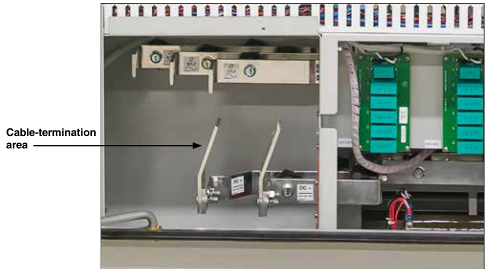
Figure 10. Cable-termination area.
