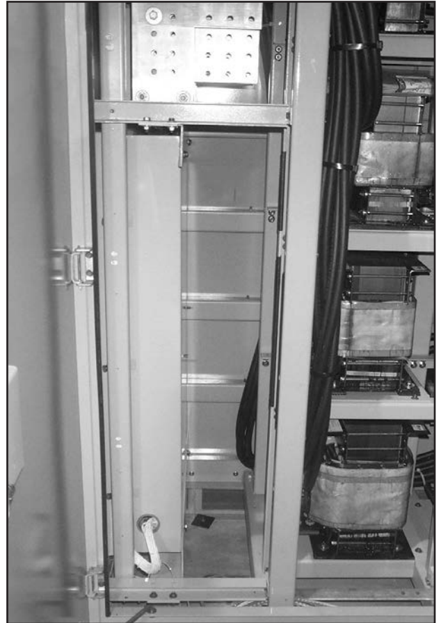
Figure 12. Control section shown with output connections for underground conduit (left). Close-up of cable entry area behind control panel (right).
