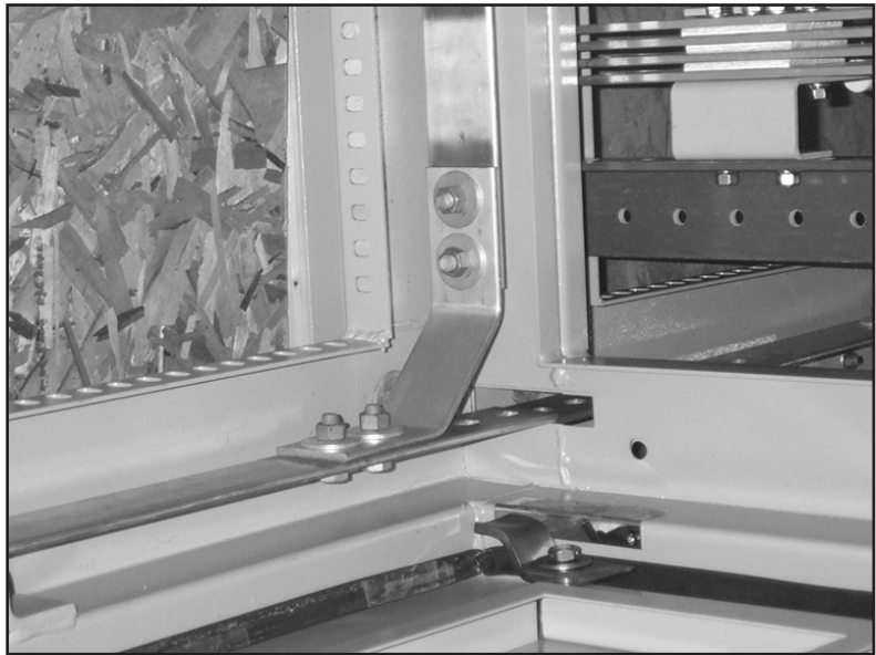
Figure 11. Attach grounding pad to facility system ground.
