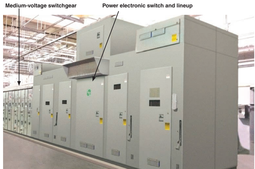
Figure 5. Medium-voltage switchgear and power electronic switch lineup for the PureWave UPS XT System.
