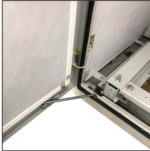
Figure 6. Lock bar at the bottom of a bay door.
