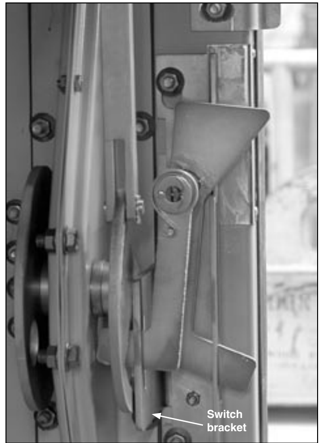
Figure 9b. Enclosure door opened—interlock engaged to the switch.
