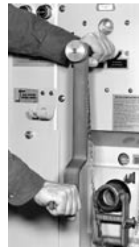
Figure 20. Dual purpose manual handle on the charging shaft.
