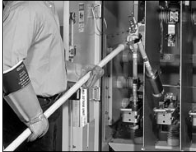
Figure 3. Installing or removing fuse using Grapp1er.
