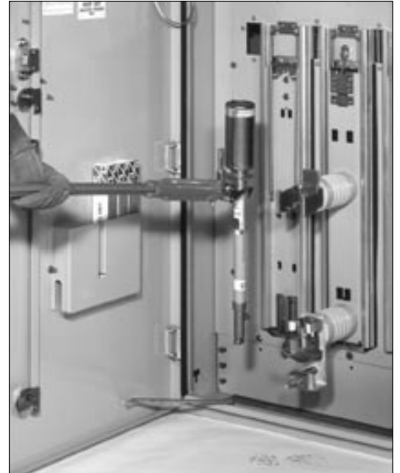
Figure 7. Installing (or removing) fuse using shotgun stick.
