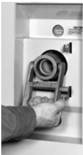
Figure 18. Decoupler handle being moved upward to decouple switch from associated switch operator.
