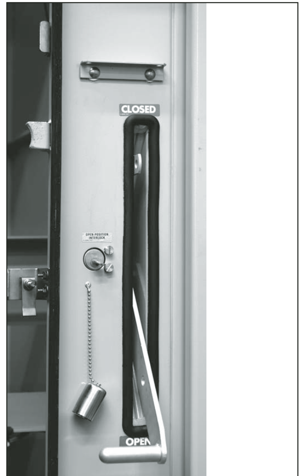
Figure 28. Key interlock.
