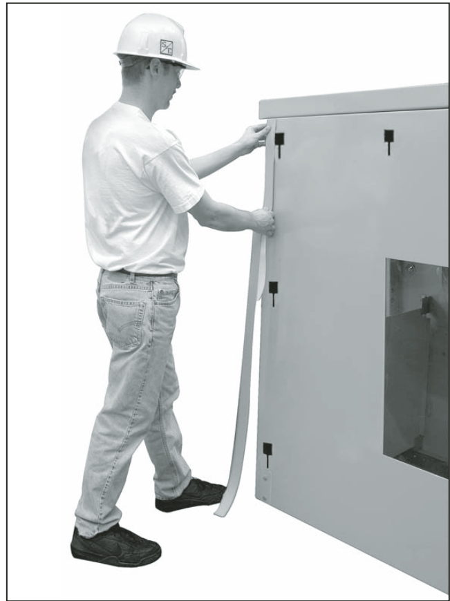
Figure 6. Apply gasketing tape \frac{1}{8} inch from edge.
