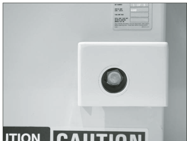
Figure 4. Pentahead bolts secure the rear access panel.
