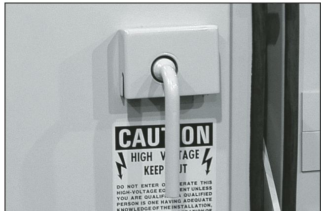
Figure 3. Non-removable manual handle—requires rotation of 90° to open or close door. Handle is padlockable. A snaplock is also pictured.
