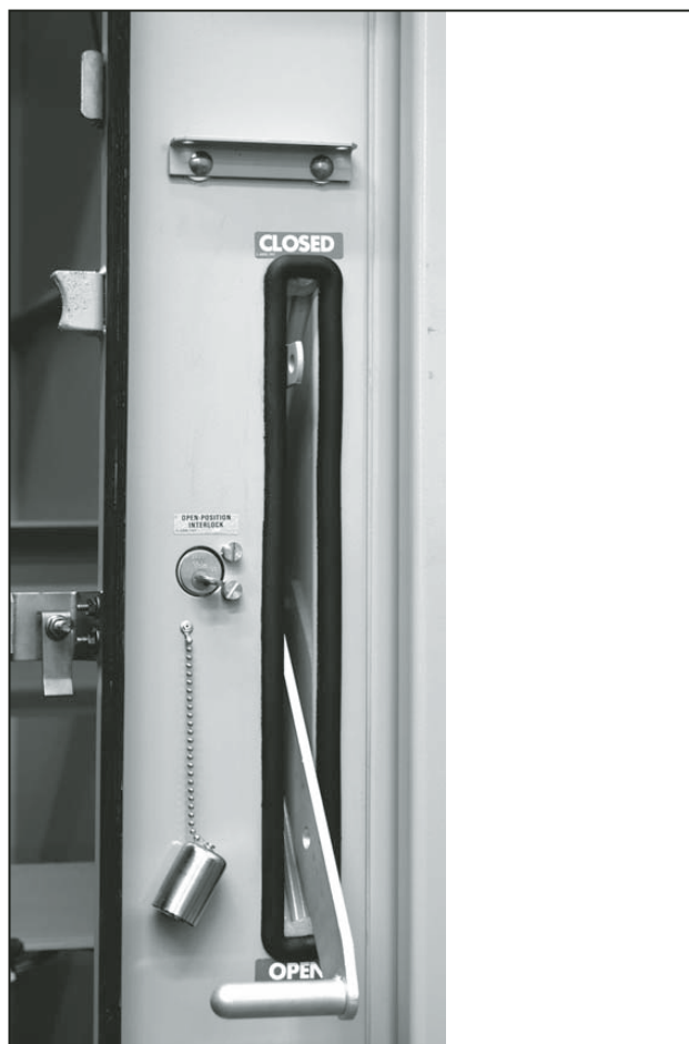
Figure 21. Key interlock.
