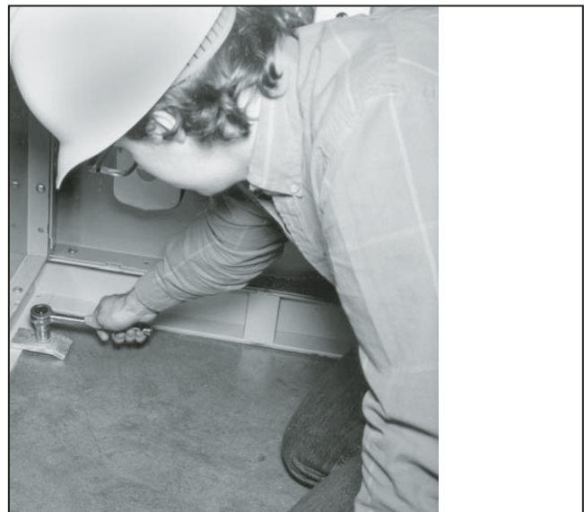
Figure 7. Installing anchor clips and nuts.
