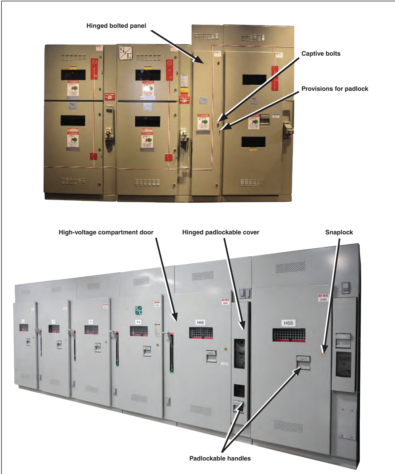
Figure 3. Two samples of switchgear showing the high-voltage compartment door, hinged padlockable cover, and hinged bolted panel.
