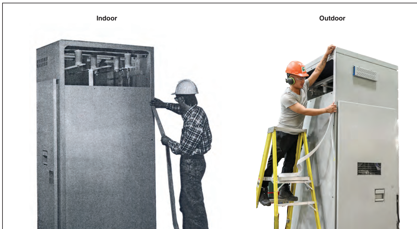
Figure 4. Applying gasket tape. Indoor units with optional dust-proof or drip-proof construction are pictured on the left. Outdoor units, pictured at right, require two strips of gasket tape at the top of the enclosure.
