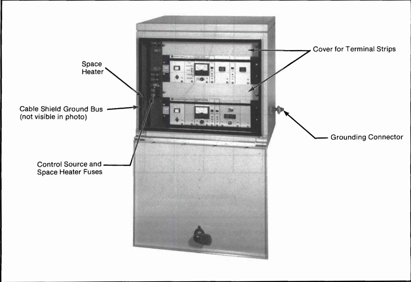
**Figure 3. S&C Automatic Control Device—Type GP/VR mounted in weatherproof enclosure.**
