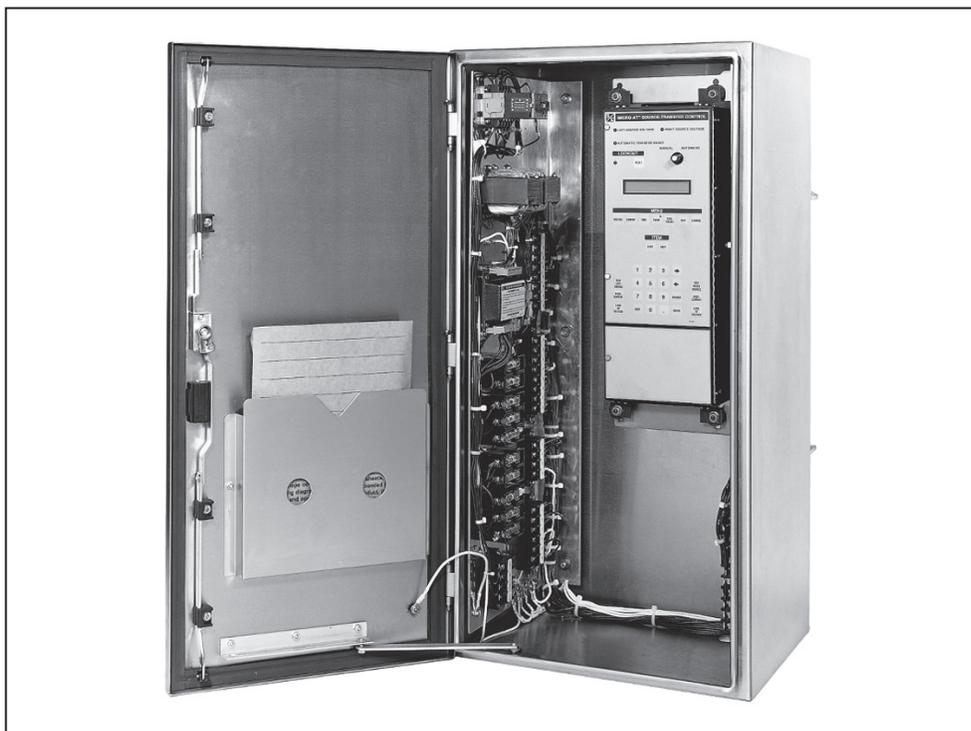
Figure 1. A Micro-AT Source-Transfer Control In a weatherproof enclosure.
