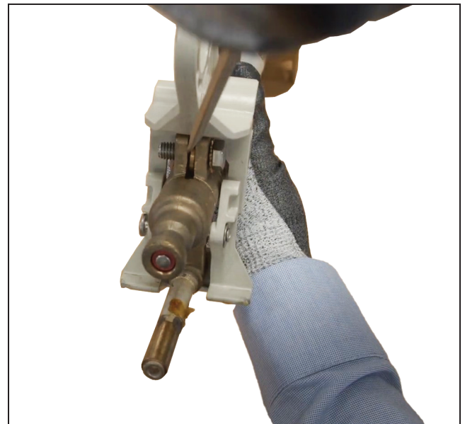
Figure 6. An SM-20 Fuse Unit upper end-fitting showing a screwdriver prying the clamp and spacer washer slightly apart, after loosening the clamp screw, as part of the fuse-replacement procedure.
