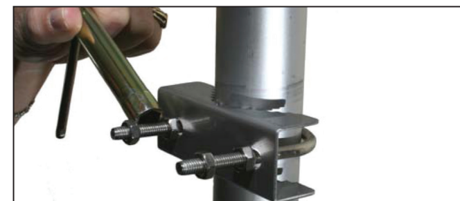
Figure 5. U-bolt mounted on pole.
