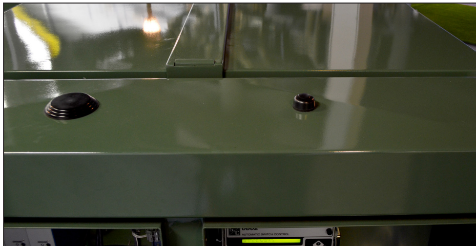
Figure 12. The left antenna is used by the SCADA radio. The dual antenna for both GPS and Wi-Fi is located at the right on this pad-mounted gear enclosure.
