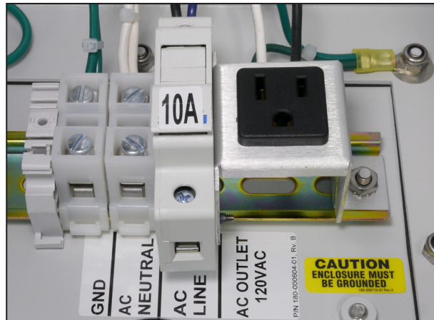
Figure 20. Connection terminal for ac control power.
