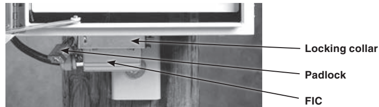
Figure 6. Bottom of switch control enclosure with the FIC connector.
