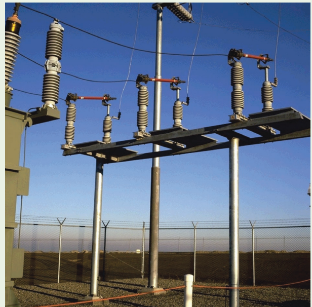
FIGURE 1. Transformer protection using SMD Power Fuses.
