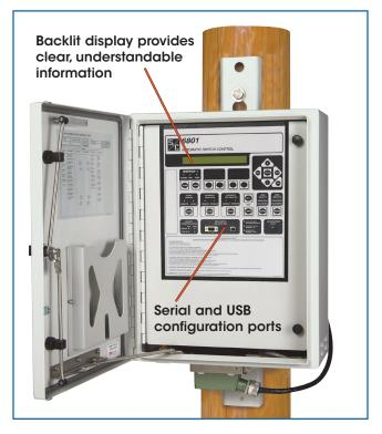
The 6801 switch control supports a variety of communication gateway hardware options and software protocols. Hardware options include:
