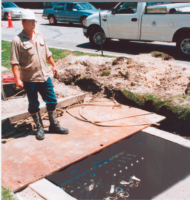
S&C installing automated distribution equipment.
