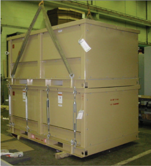
Two units of the airworthy Vista switchgear can be stacked to save space. Turnbuckles attach to heavy-duty eye bolts to hold the units together during transport.
