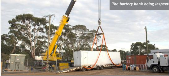
Crews install the containerized PureWave $^{ extsf{R}}$  SMS Storage Management System.
