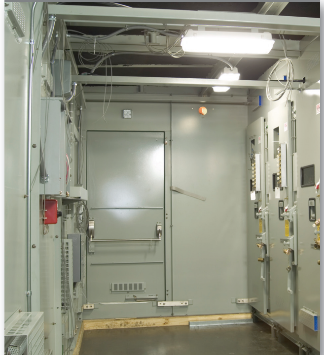
Inside view of the airport seven-bay lineup.
