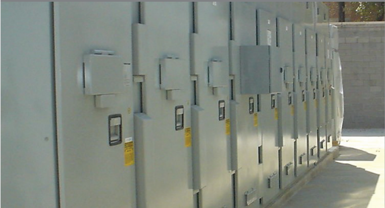
Installed custom metal-enclosed switchgear
