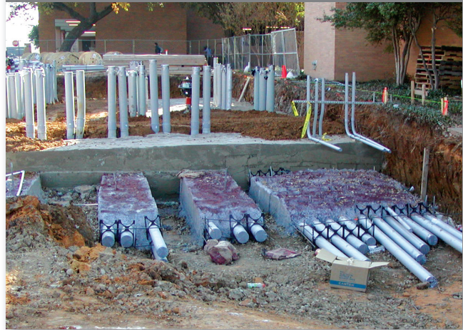
Groundwork for custom metal-enclosed switchgear
