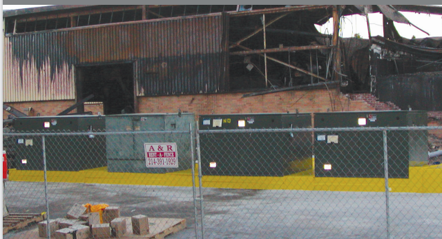
Consigned S&C Pad-Mounted Gear
