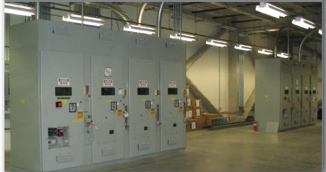
Four-bay lineups of 15-kV switchgear.
