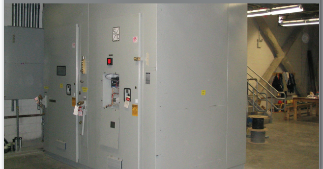
Two-bay lineups of 38-kV switchgear.
