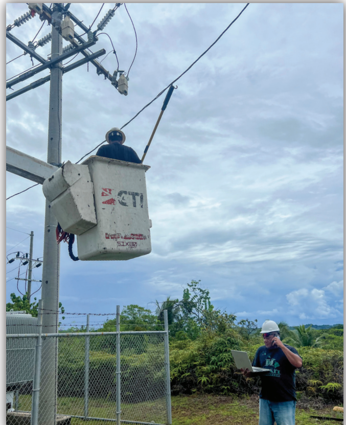
FIGURE 3. TripSaver II reclosers installed on PPUC's network.
