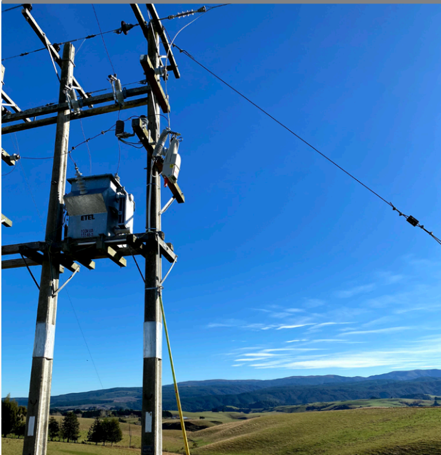
A TripSaver II recloser protects SWER lines in New Zealand.
