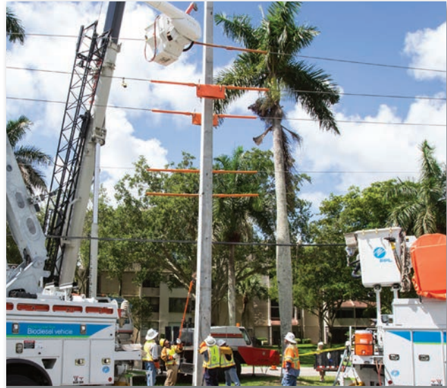
Wooden poles are replaced with concrete poles.
