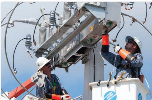
An IntelliRupter fault interrupter being installed.
