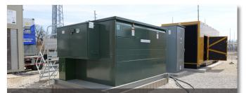
Figure 2. The Remote Supervisory Vista Underground Distribution Switchgear connects the various systems.
