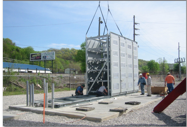
Installation of battery rack.
