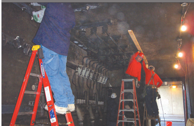
Shortly after construction started.
