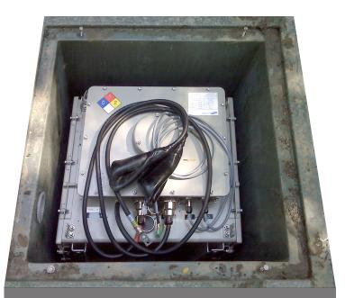
A Li-lon battery being placed in an underground vault, beneath S&C's PureWave® CES unit.
