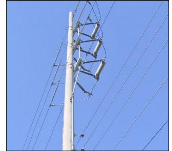
Line-Rupter™ Switch
