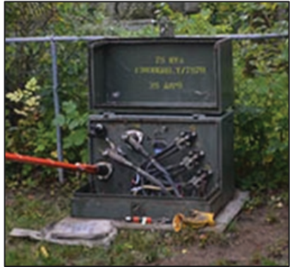
EdgeRestore® Underground Distribution Restoration System
