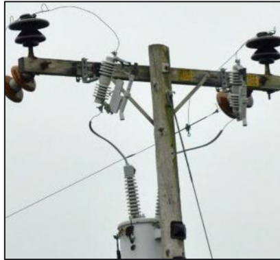
Fault Tamer® Fuse Limiter
