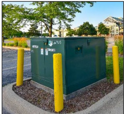
PMH Pad-Mounted Gear
