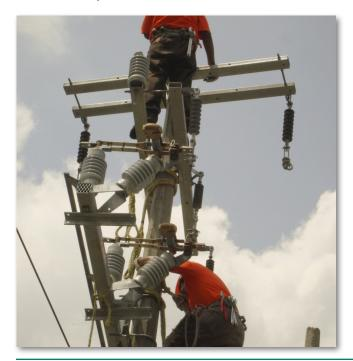
This type of switch, which is renown for its rugged construction and reliability, is specifically designed to perform live switching duties. The switch was easily installed by CFE-certified personnel hired by CPIngredientes.
