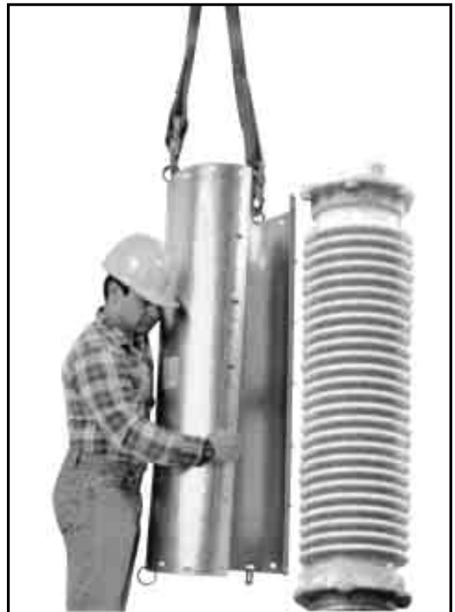
Figure 2. Raising spare interrupter container into position on interrupter being replaced. Model 2030 Circuit-Switcher illustrated; Models 2020 and 2025 are similar.
