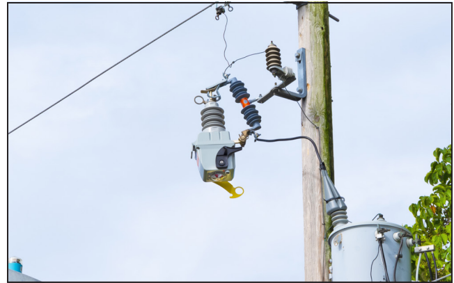
S&C's VacuFuse Self-Resetting Interrupter.
