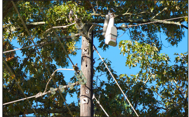
S&C's TripSaver II Cutout-Mounted Recloser.
