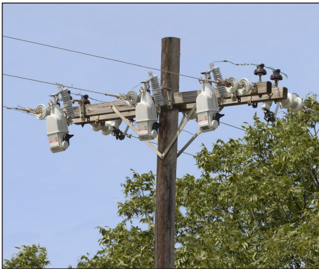
S&C's TripSaver II Cutout-Mounted Recloser in three-phase, group operations configuration.
